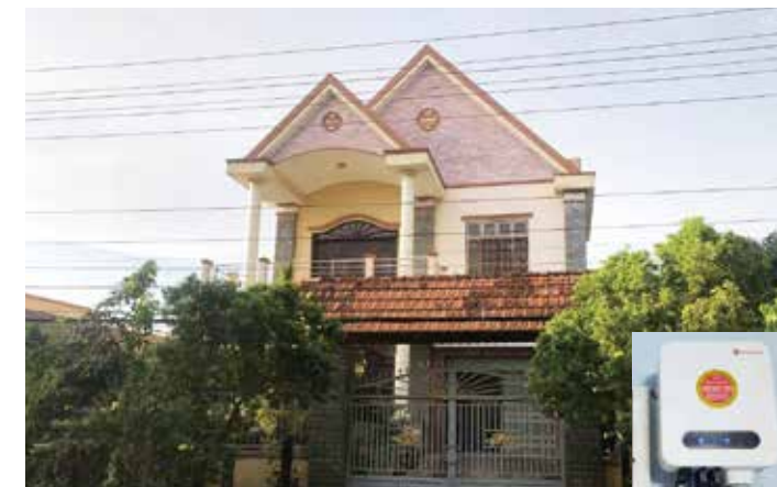
Residential PV Project in Vietnam
